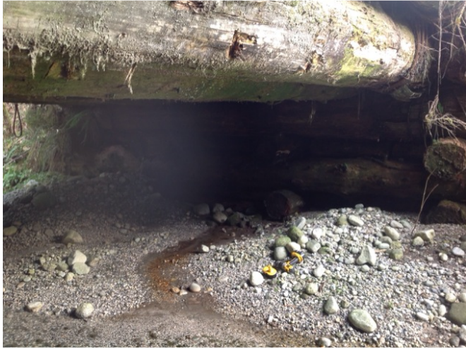
Left Bank Abutment when facing downstream
