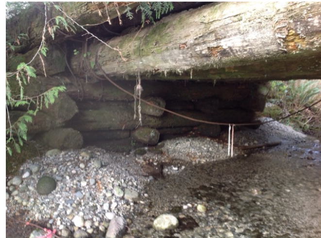
Right Bank Abutment when facing downstream
